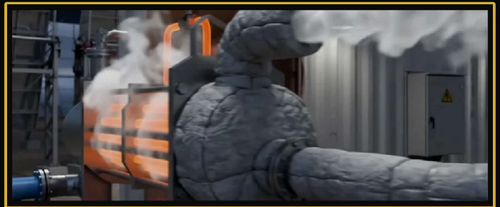
04 The heated liquid is pumped through an exchanger to create a pressurized vapor.
