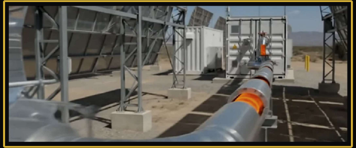
02 The heated liquid is pumped into insulated chambers.
