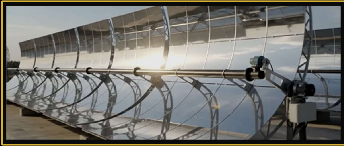
01 Sunlight hits parabolic troughs, focusing on the center pipe and heating the liquid inside.
